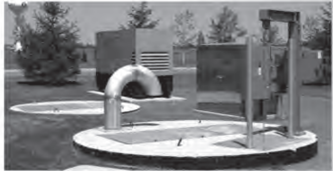
Lift Stations-New and Retro-fit Upgrades
