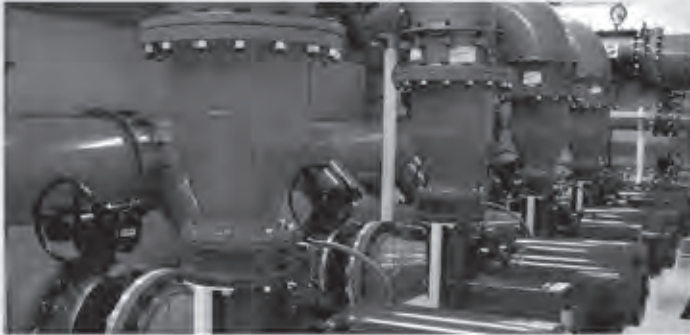
Booster Pump Stations
