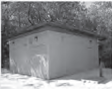
Housed Pump Systems
